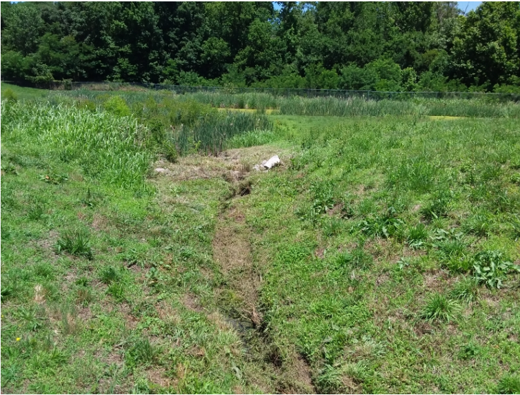
BMP 30- erosion occurring throughout inlet channel
