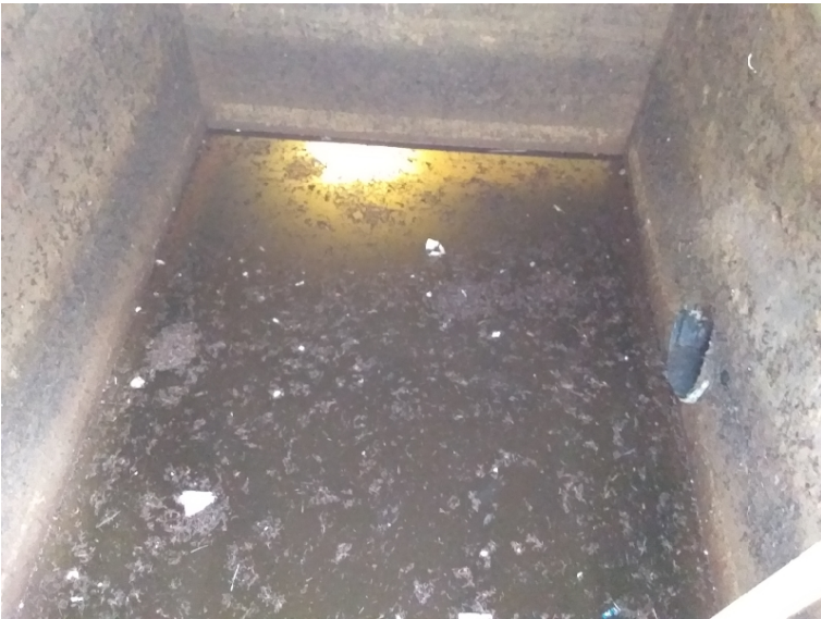
BMP 27- trace amounts of sediment and minor trash
