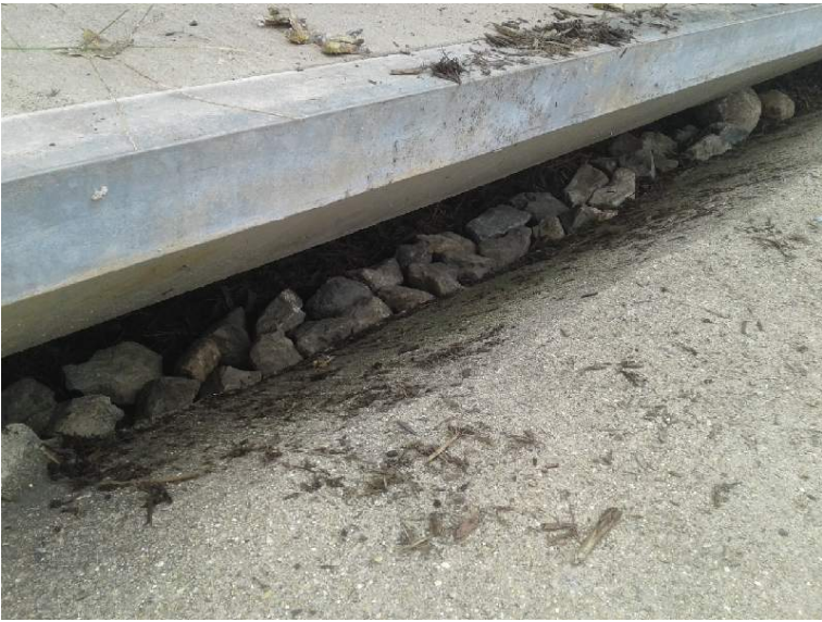
Unit 41: after 2 rows of inlet stones installed
