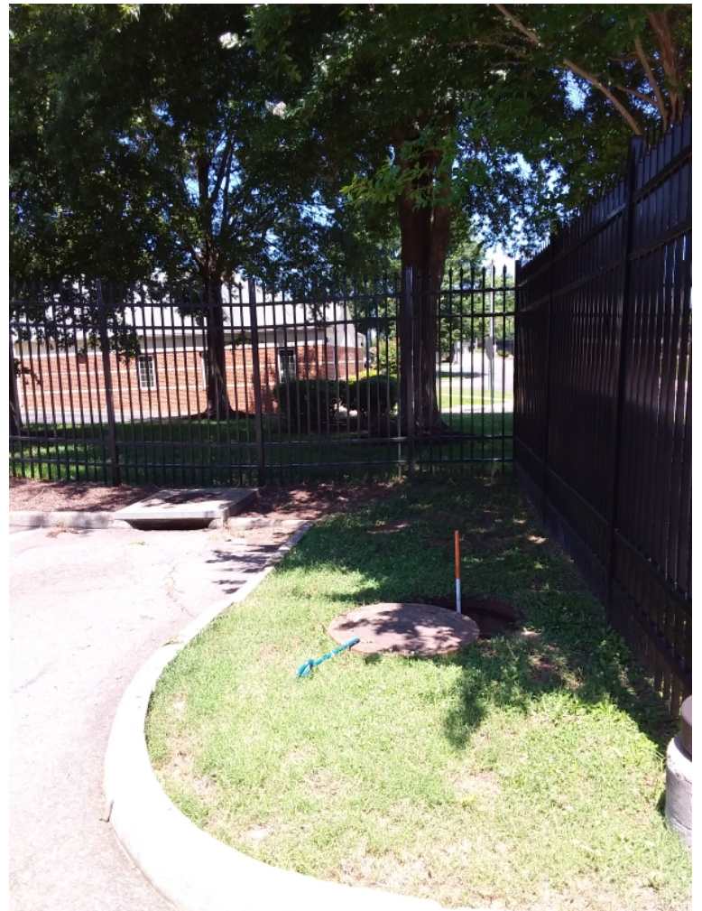
BMP 33- recycle trash can was sitting on top of lid and had to be uncovered with 2" of mulch on top of entire manhole lid
