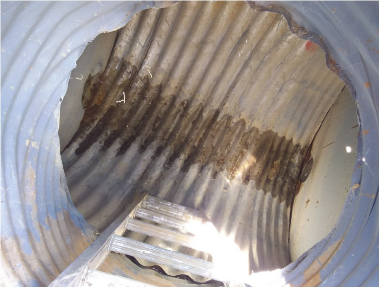
BMP 26: no significant sediment, trash or debris
