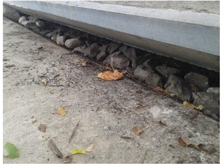
Unit 8: After 2 row inlet stones installed
