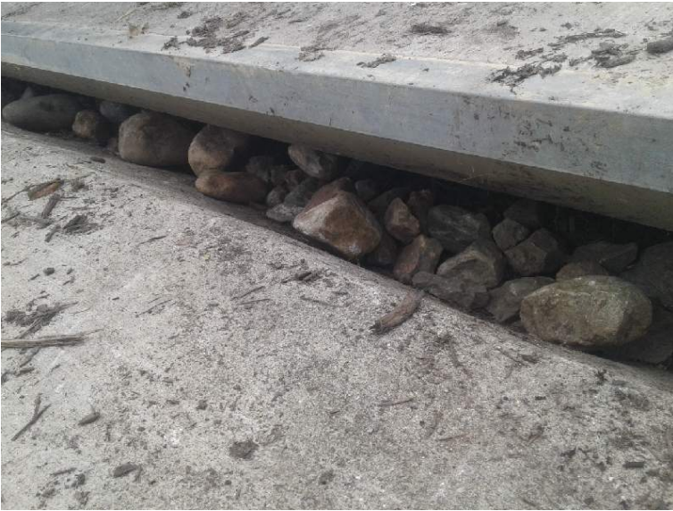
Unit 42: after 2 rows of inlet stones installed
