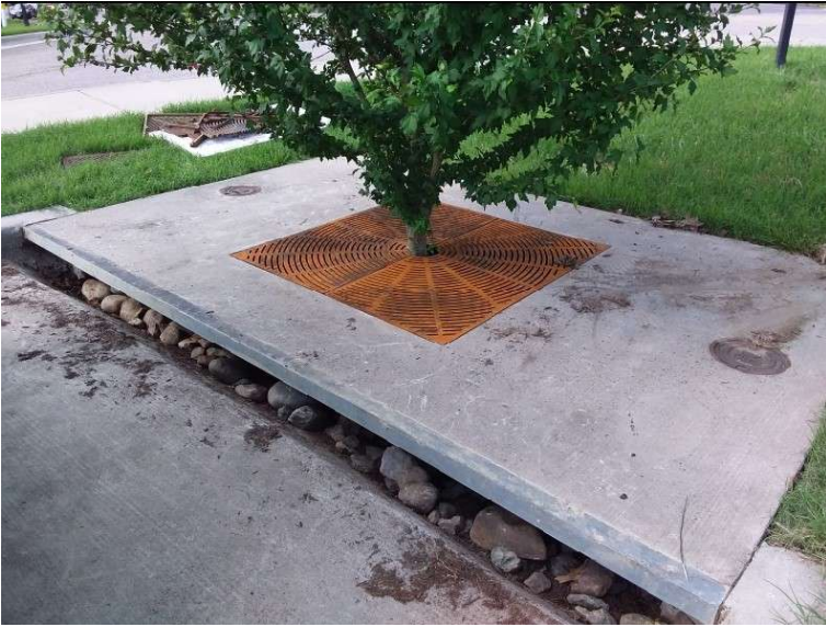
BMP 42 Grate replaced
