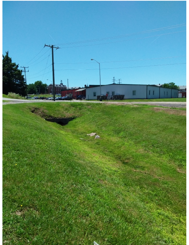
BMP 30- inlet channel
