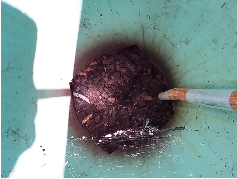
BMP 38- minimal sediment and gravel found in maintenance port
