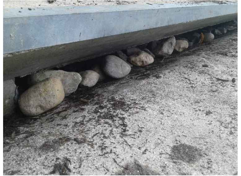
Unit 9: after 2 rows inlet stones installed.
