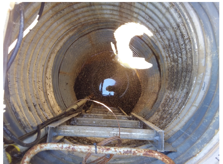
BMP 24: 7' of water and minimal sediment
