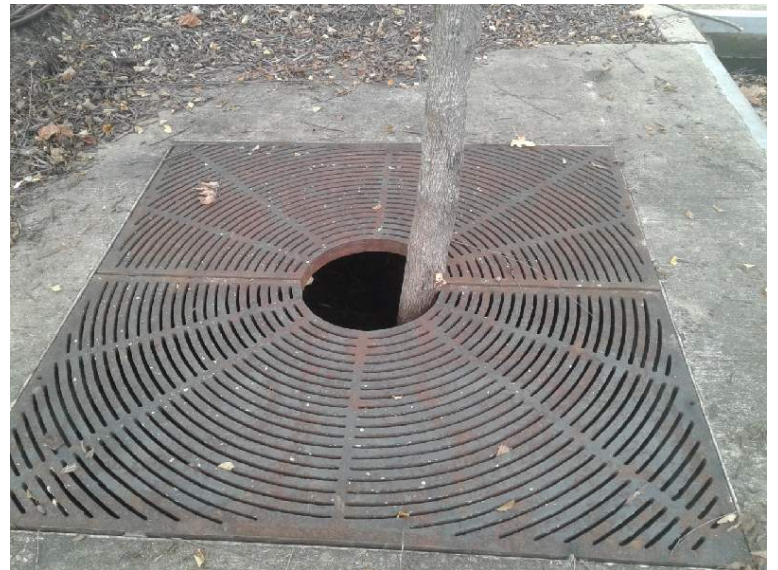
8: tree is growing over grate
