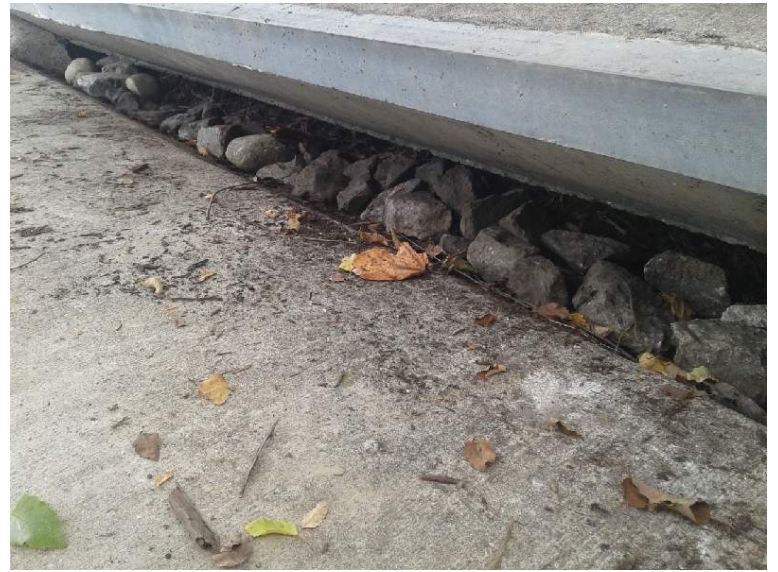
Unit 12: After, 2 rows of inlet stones installed
