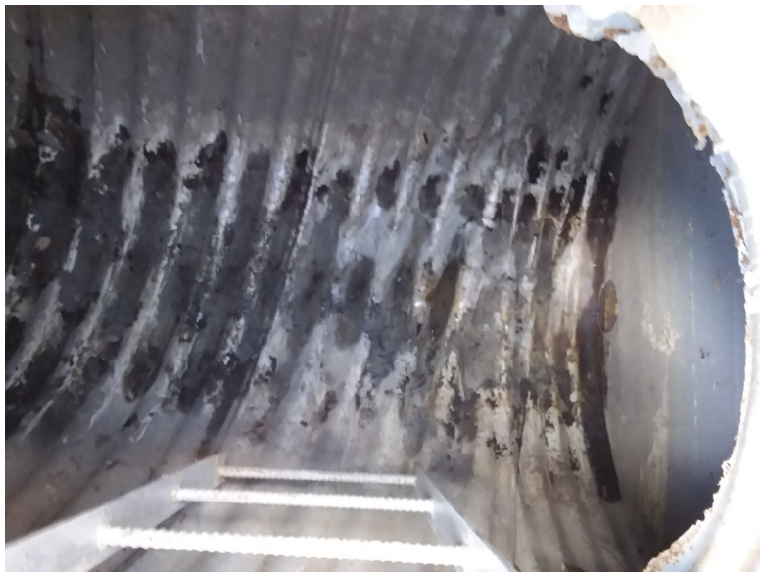
BMP 40- all floatables, debris, and sediment removed
