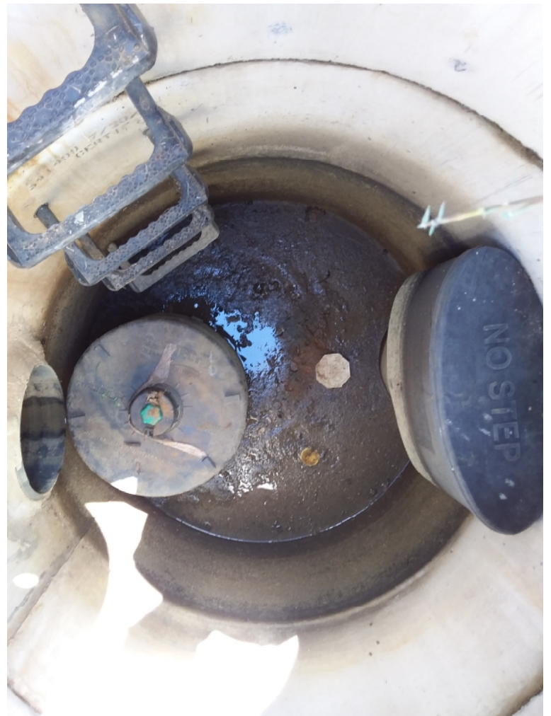
BMP 23: minimal sediment accumulation
