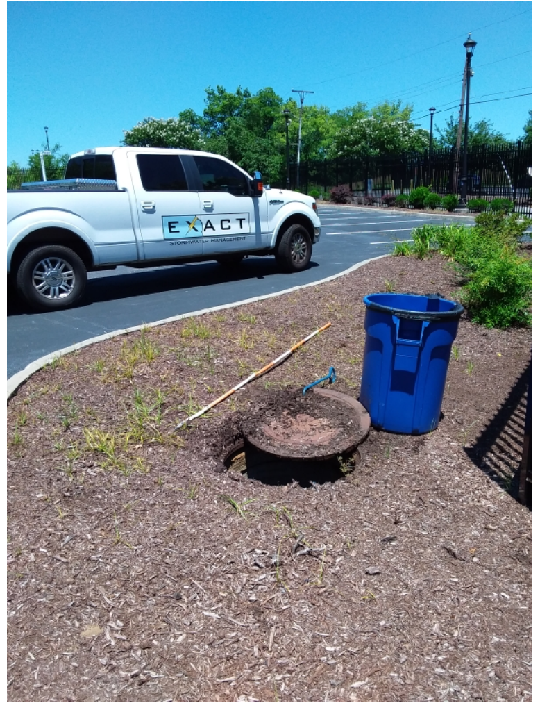
BMP 33- recycle trash can was sitting on top of lid and had to be uncovered with 2" of mulch on top of entire manhole lid
