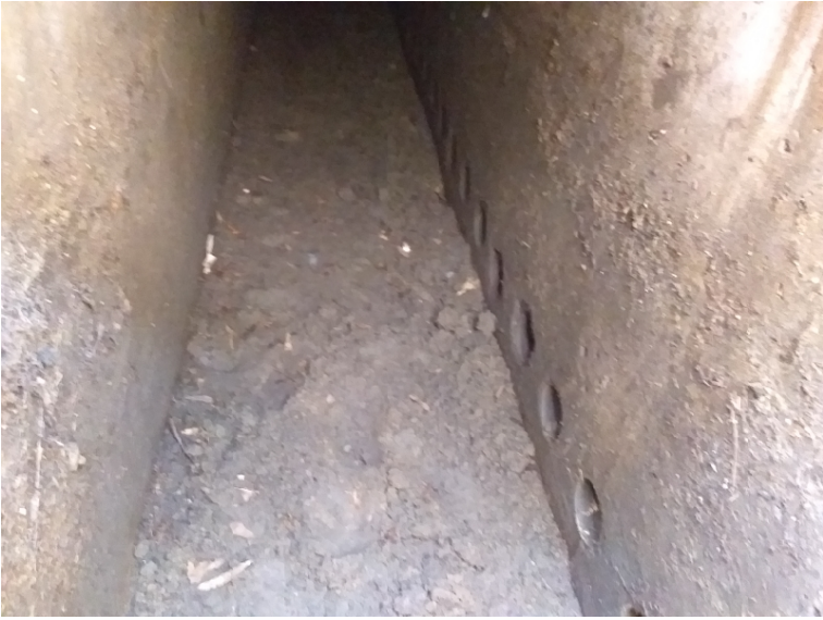
BMP 31: sand filter side- no sediment noted
