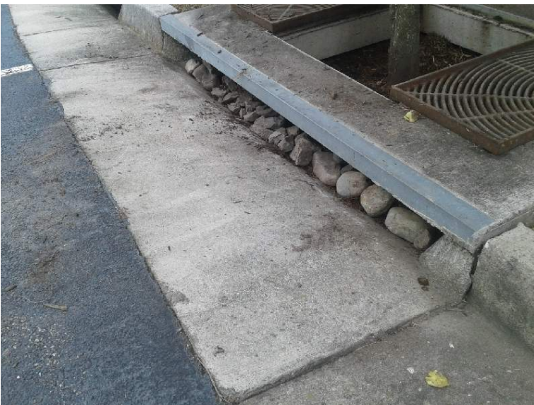
Unit 13: After 2 rows of inlet stones installed.
