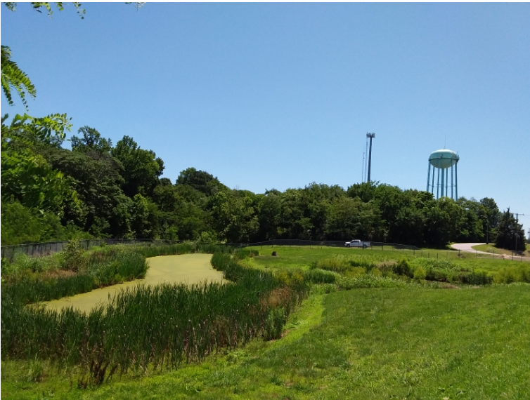
BMP 30- cattails along the aquatic bench surrounding the entire pond and duck weed has taken over the surface water
