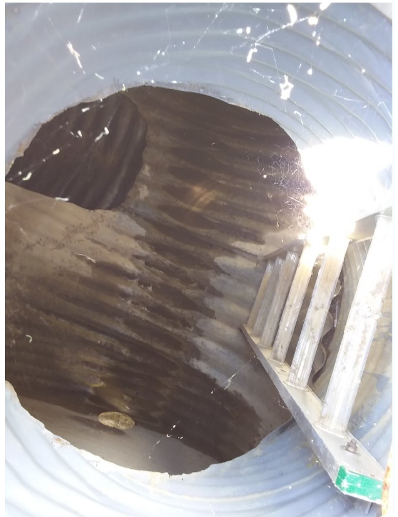
BMP 26: no significant sediment, trash or debris
