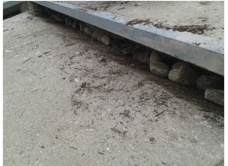
Unit 43: After 2 rows inlet stones installed
