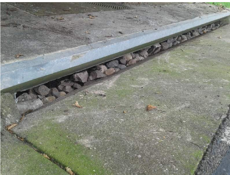
Unit 10: After 2 rows of inlet stones installed.
