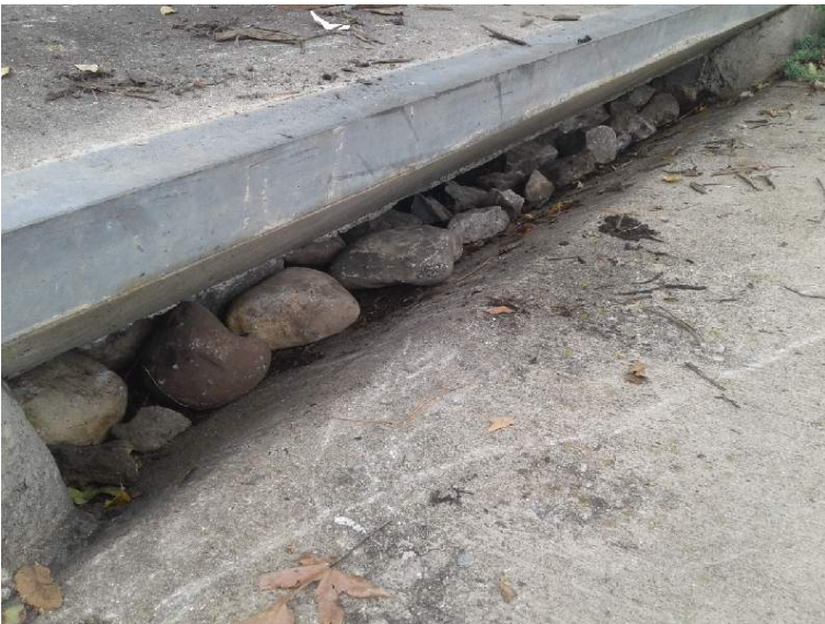
Unit 7: after 2 rows Inlet stones installed
