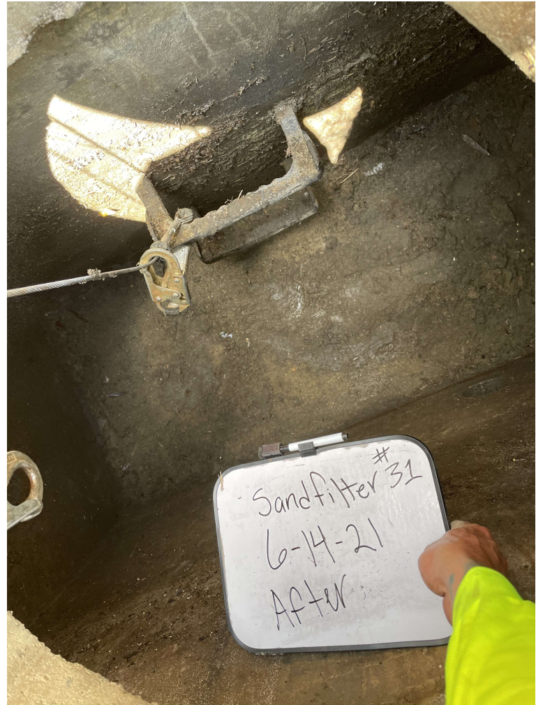
BMP 31 Sandfilter After
