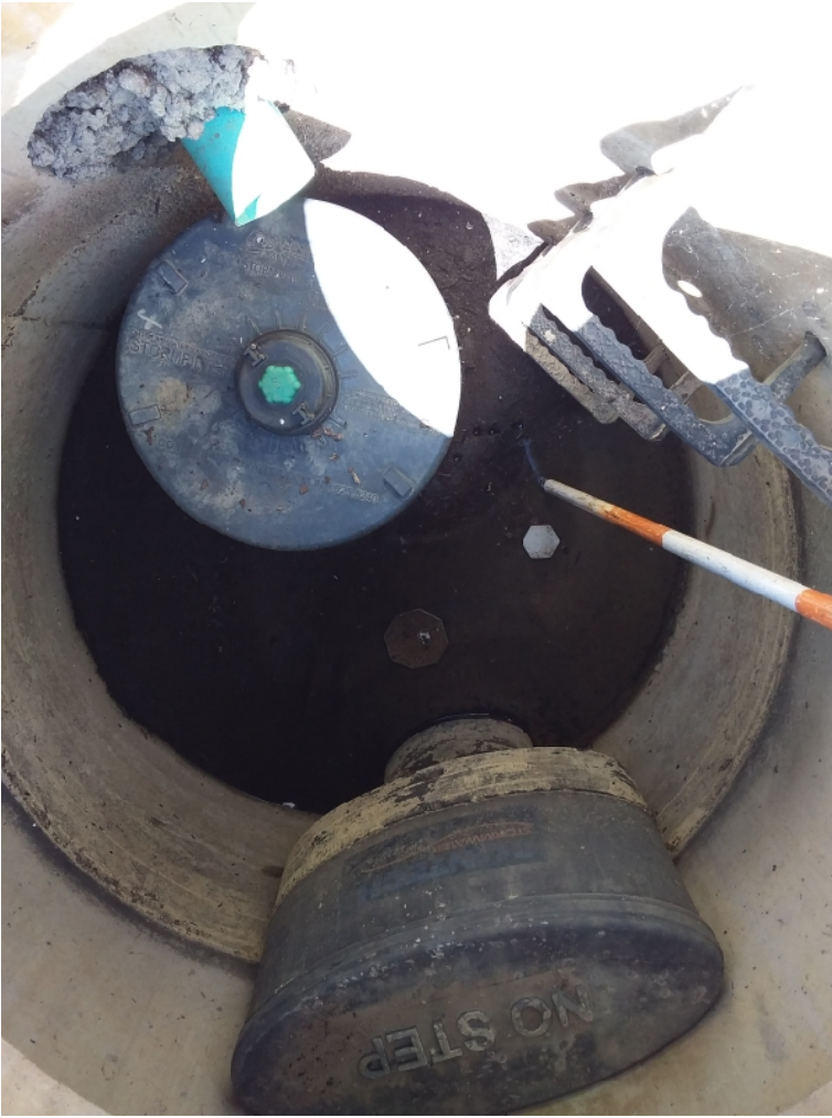
BMP 22- remove accumulated sediment for next maintenance visit
