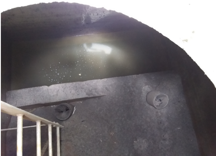
BMP 28- dewater chamber and remove from far side of weir wall
