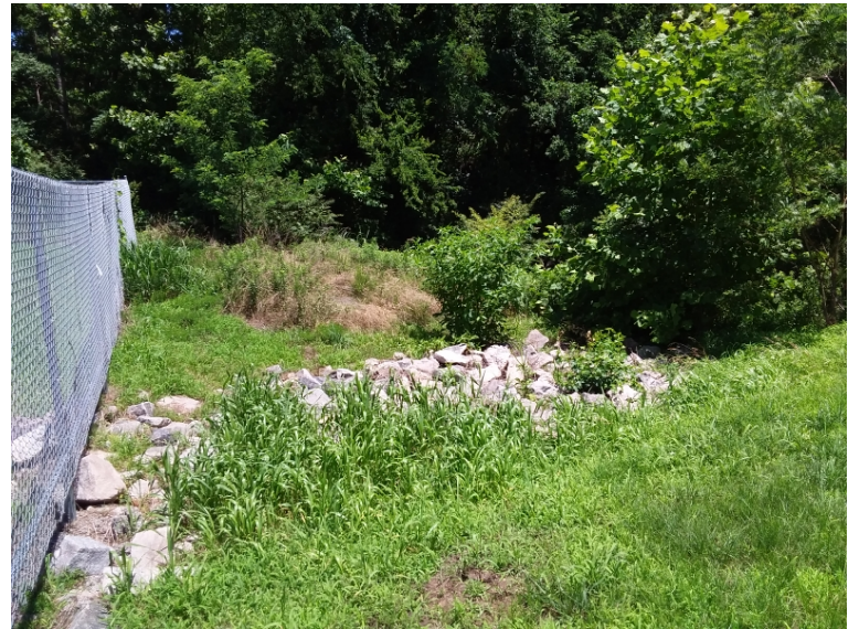
BMP 30- emergency spillway
