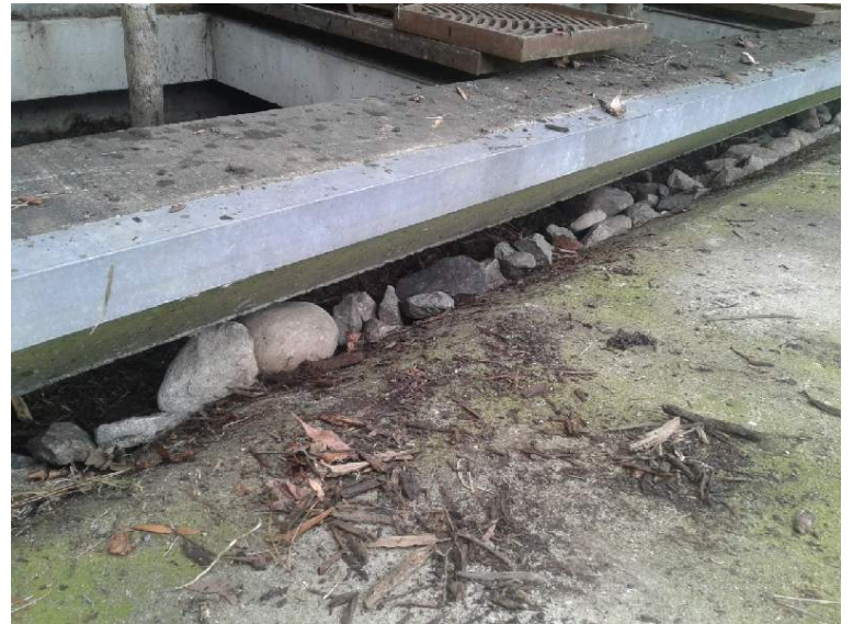
Unit 10: After 2 rows of inlet stones installed.
