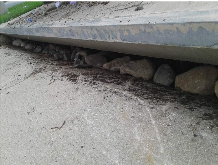
Unit 44: after 2 rows inlet stones installed
