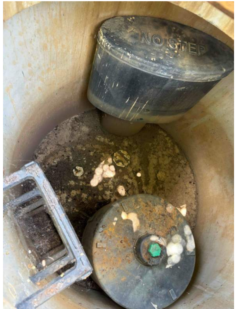
BMP 35- inside view
