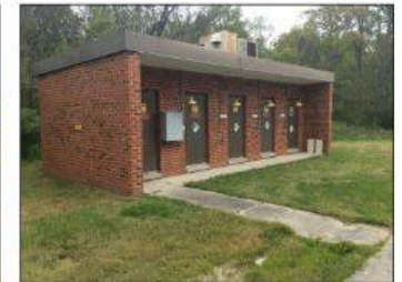
18: Hazardous Waste Storage Area
