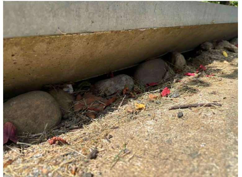
BMP 13- inlet throat after maintenance
