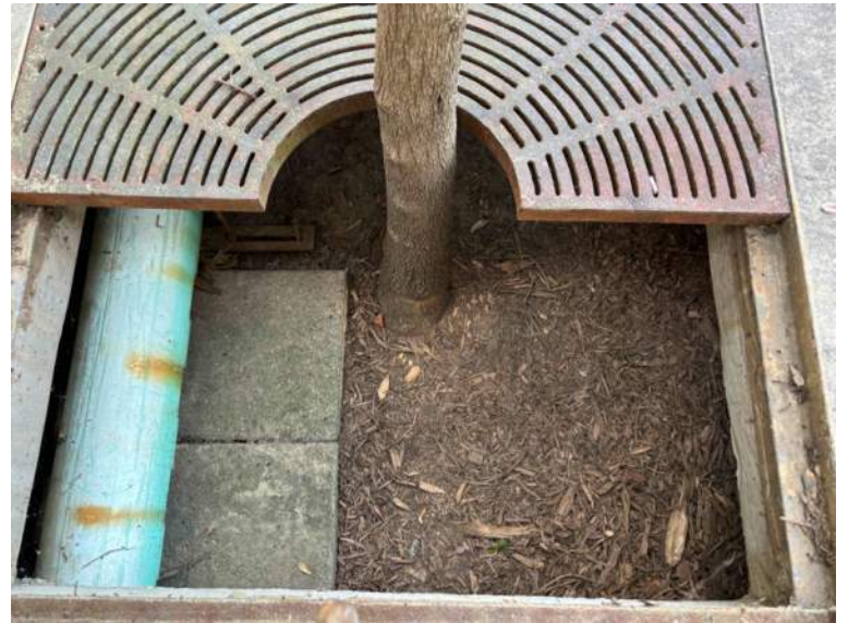
BMP 5- inside view
