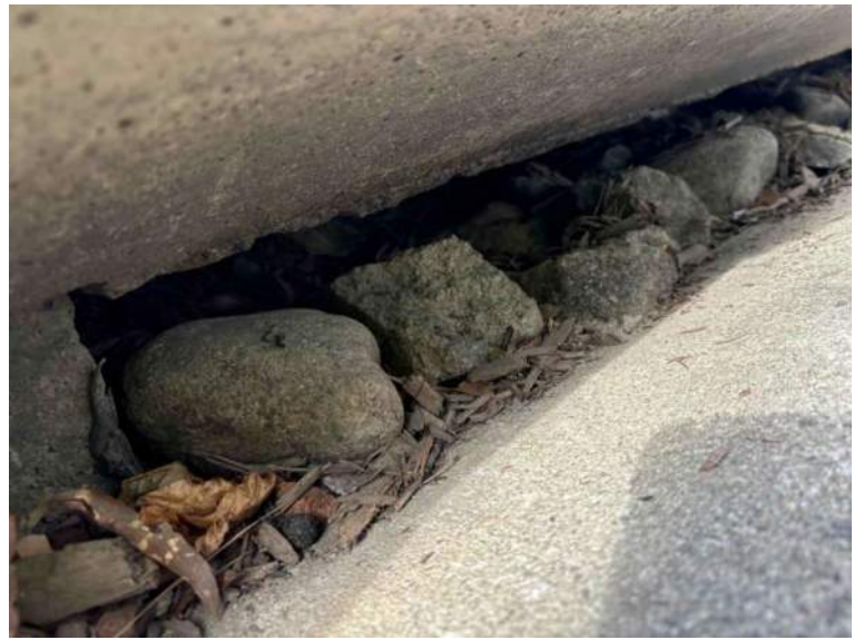
BMP 9- inlet throat after maintenance
