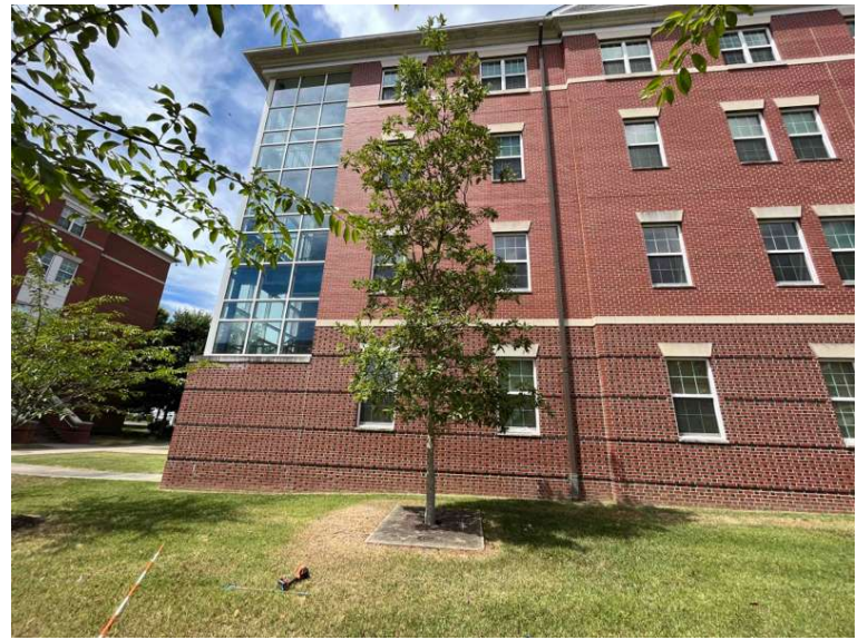
BMP 18- overall after maintenance
