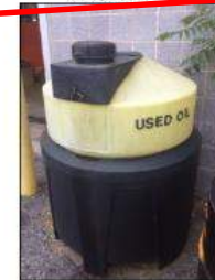
3: Used Oil Storage
