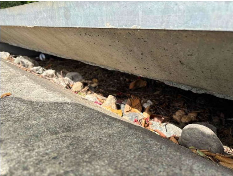
BMP 12- inlet throat after maintenance
