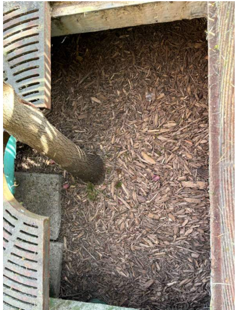
BMP 1- inside view
