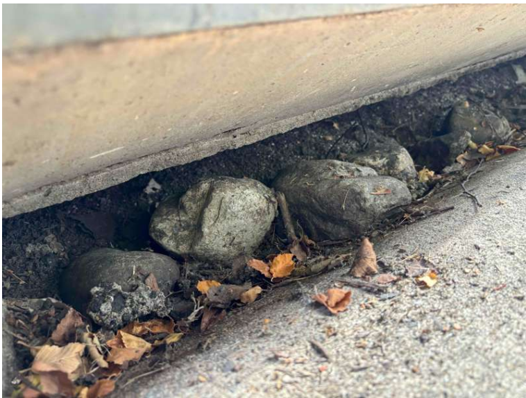
BMP 8- inlet throat after maintenance
