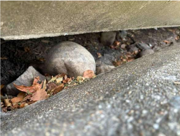
BMP 10- inlet throat after maintenance
