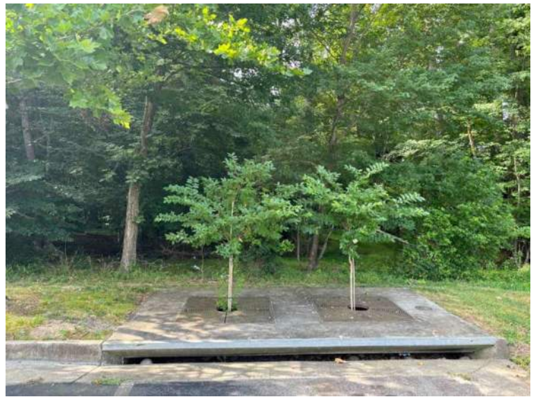
BMP 10- overall after maintenance
