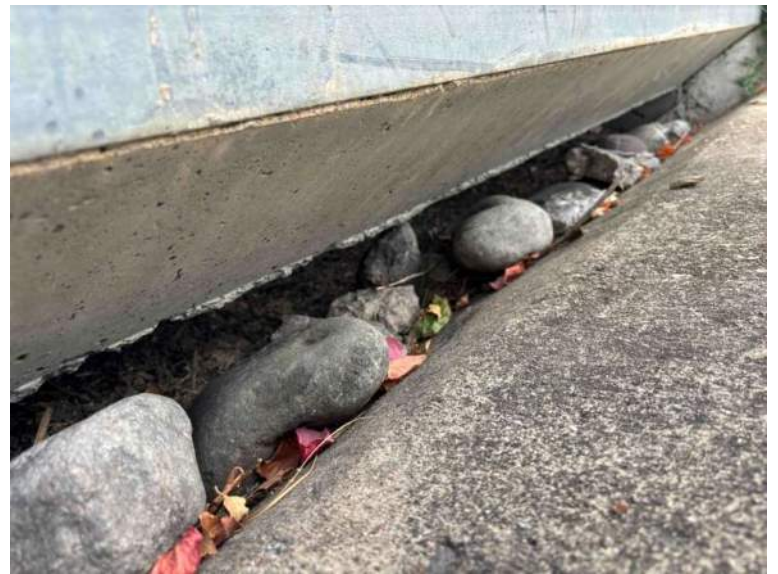
BMP 7- inlet throat after maintenance
