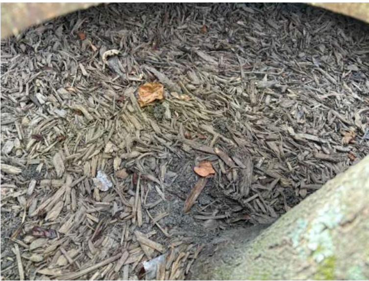
BMP 9- inside view after maintenance
