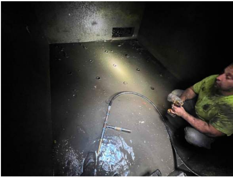
BMP 49 - after cleaning vault
