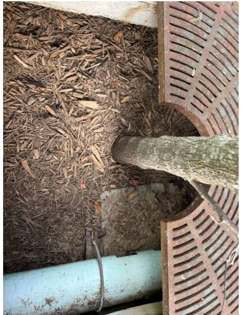
BMP 6- Inside view
