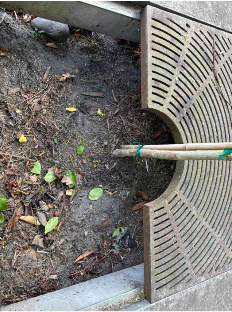
BMP 11- right inside view after maintenance
