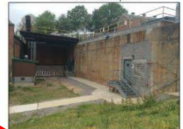
12: Heating Plant (boiler backup fuel storage)
