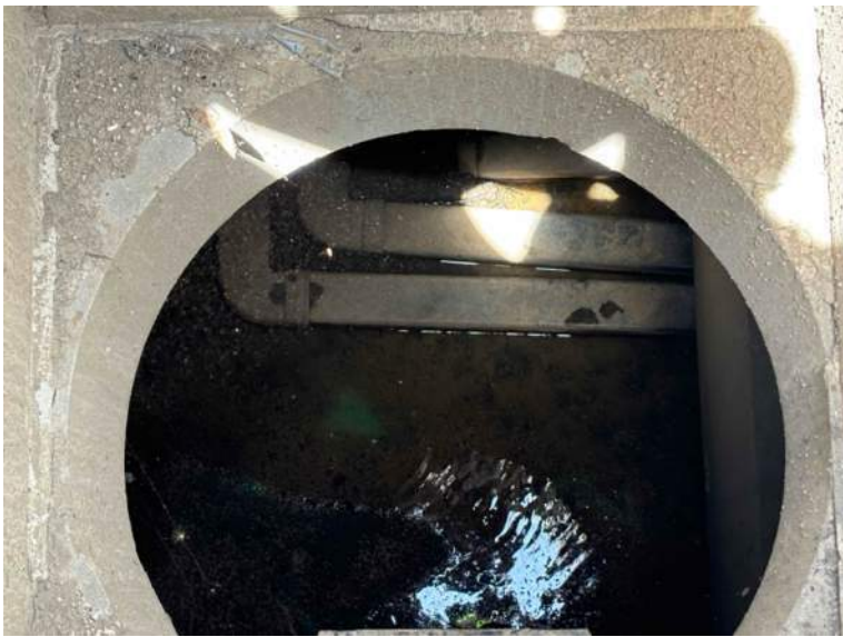
BMP 47- Outlet chamber
