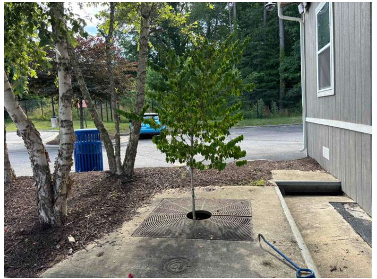
BMP 8- overall after maintenance
