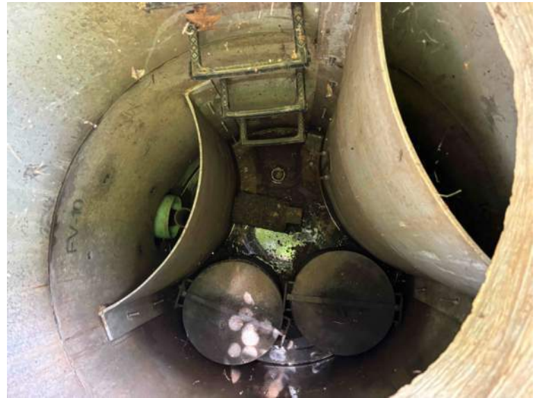
BMP 34- inside view
