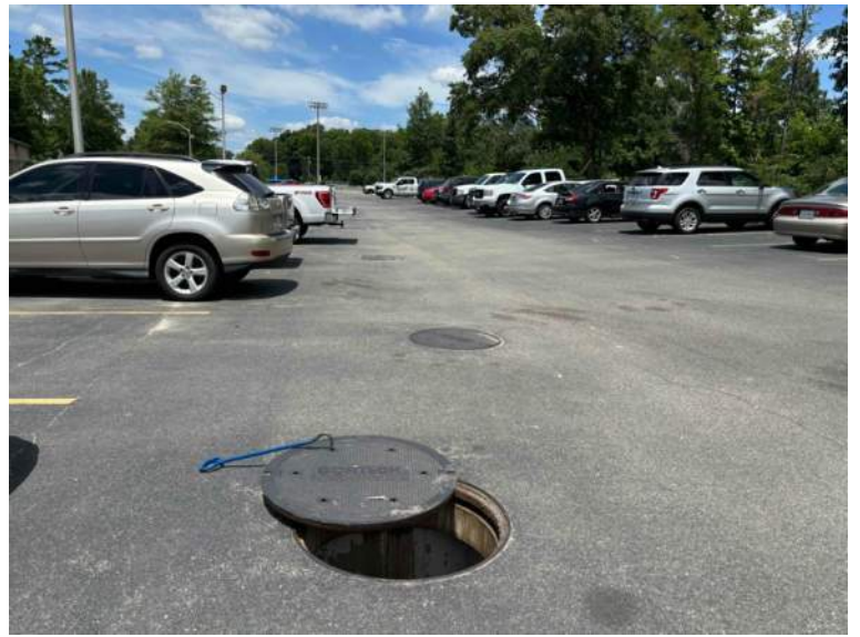
BMP 47- Outlet access
