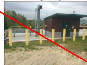
11: Heating Plant (boiler backup fuel storage)
