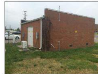
17: Hazardous Waste Storage Area
