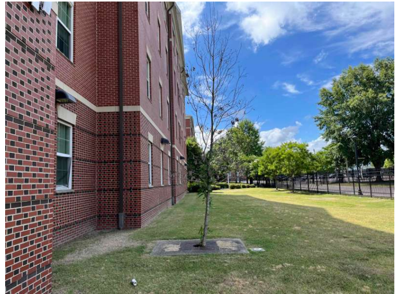
BMP 17- overall after maintenance
