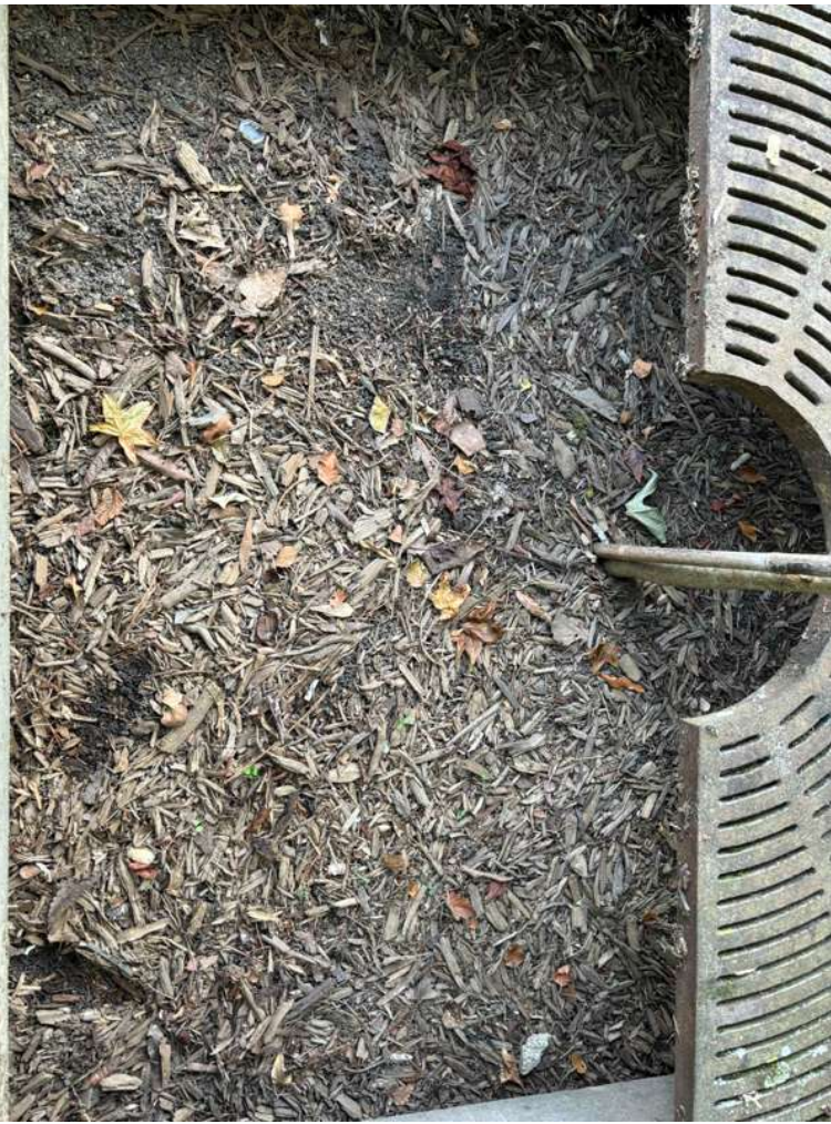
BMP 10- right inside view after maintenance
