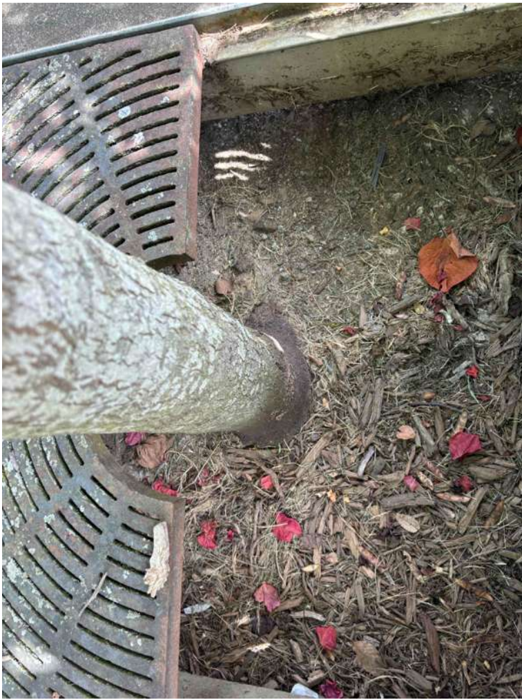
BMP 13- inside view after maintenance
