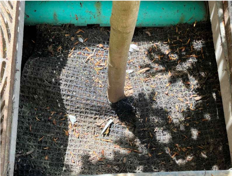
BMP 19- inside view after maintenance
