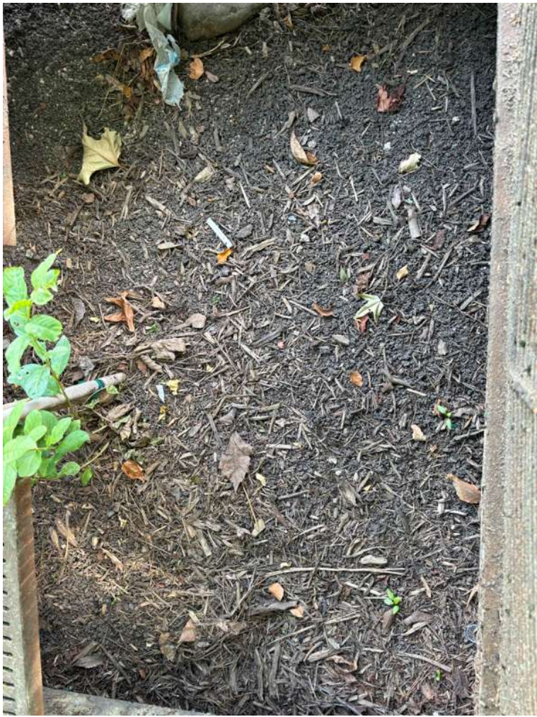
BMP 10- left inside view after maintenance
