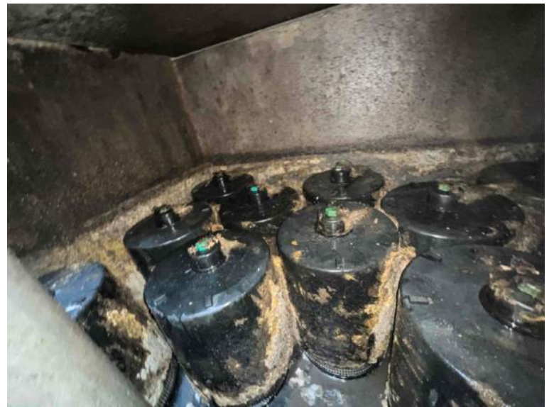
BMP 48- before replacing cartridges
