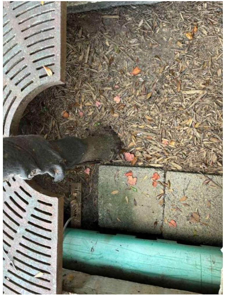
BMP 4- inside view after maintenance
