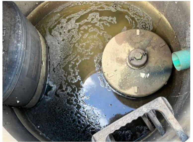
BMP 22- inside view
