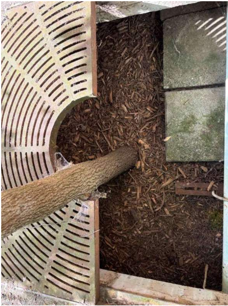
BMP 5- inside view after maintenance
