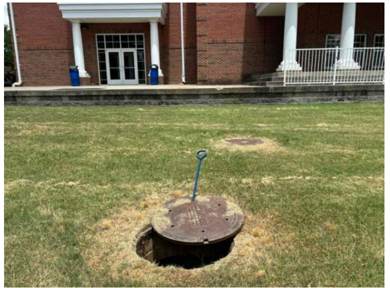
BMP 49- overall view of outlet
