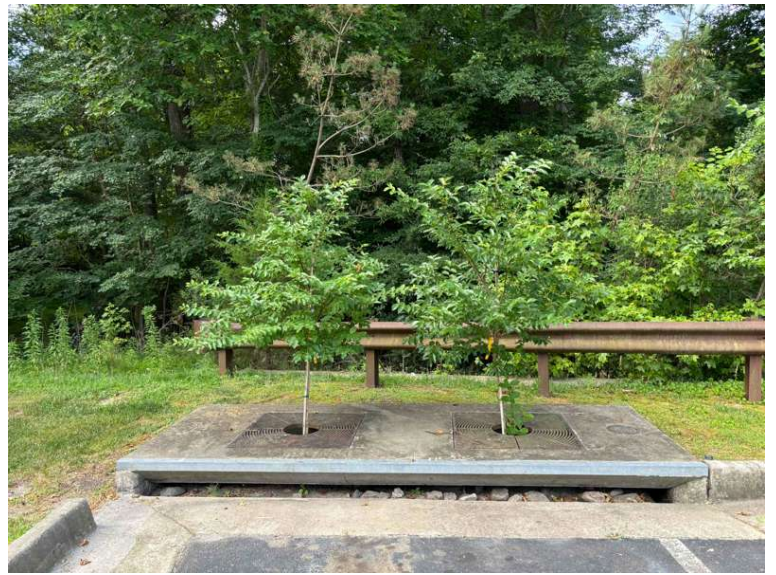
BMP 11- overall after maintenance
