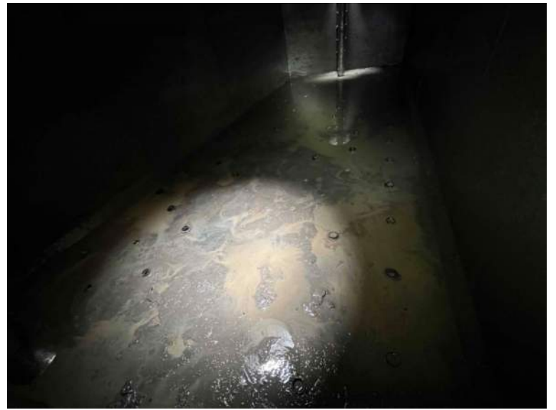
BMP 47 - after cleaning vault
