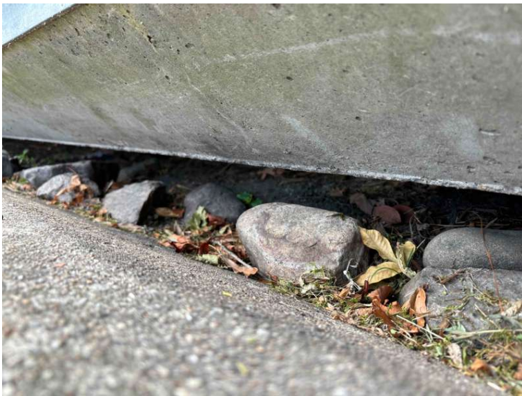
BMP 11- inlet throat after maintenance
