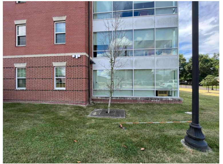
BMP 16- overall after maintenance
