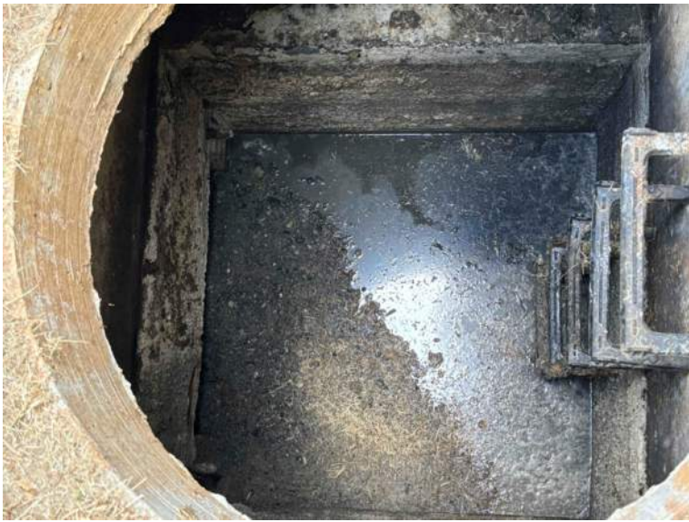
BMP 48- Inside view of outlet chamber
