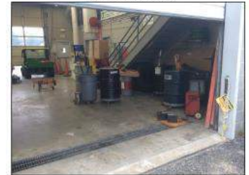
4: Maintenance Bay (with trench drain)
