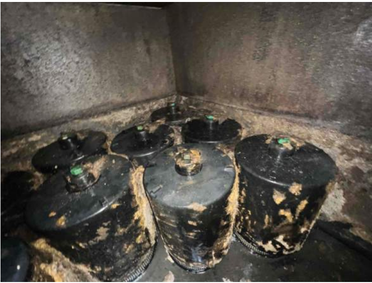
BMP 48- before replacing cartridges
