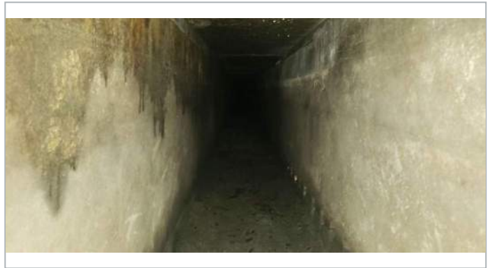
BMP 31 Progressing through the sand filter
