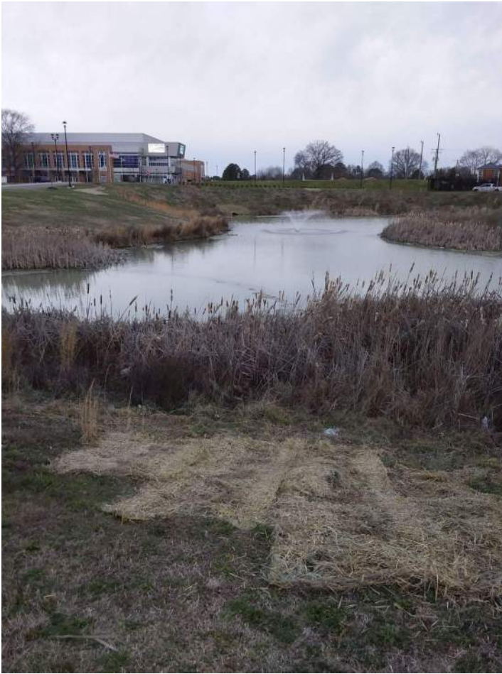
BMP 46: Bank erosion repaired with topsoil and seed and straw matting
