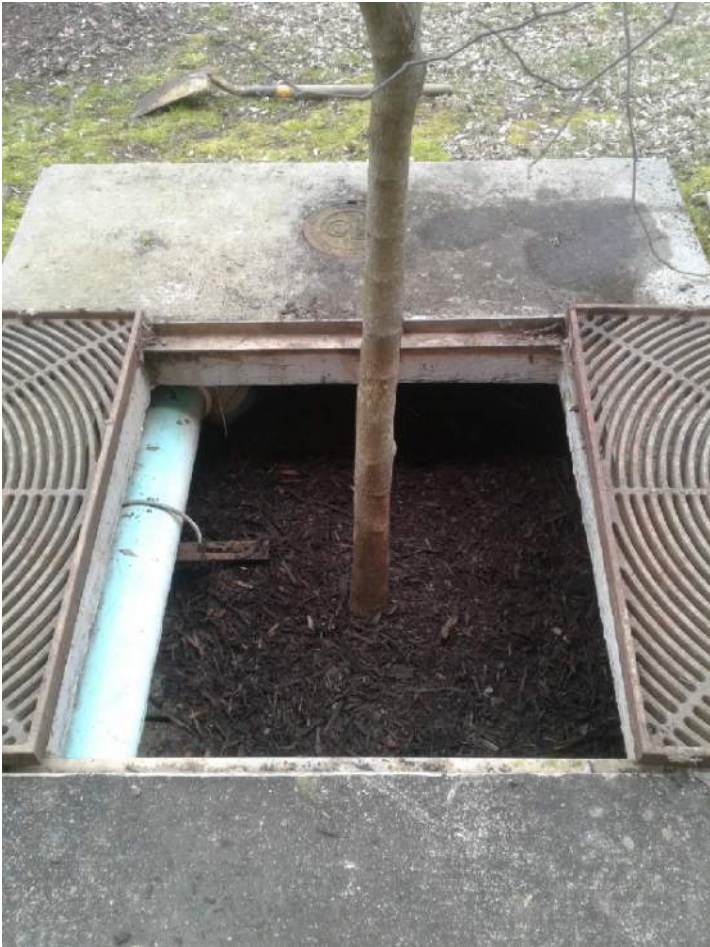
Unit 19 tree replaced and unit maintenance complete. Added media to replace lost during tree replacement.
