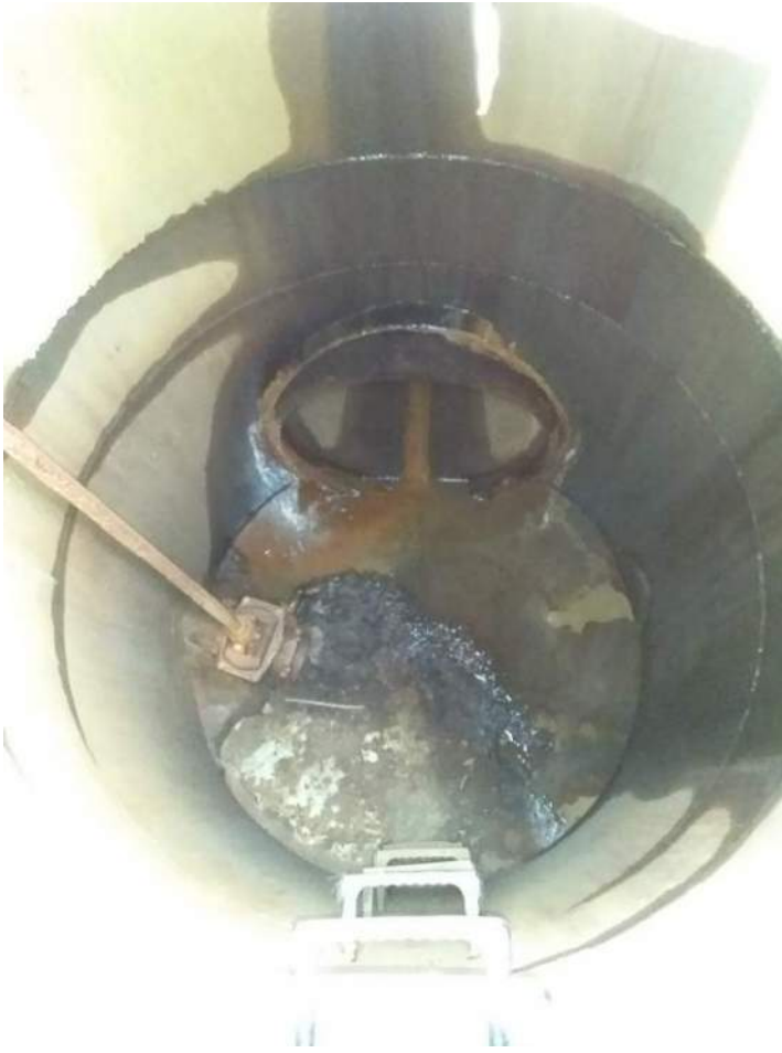
BMP 30: view under manhole
