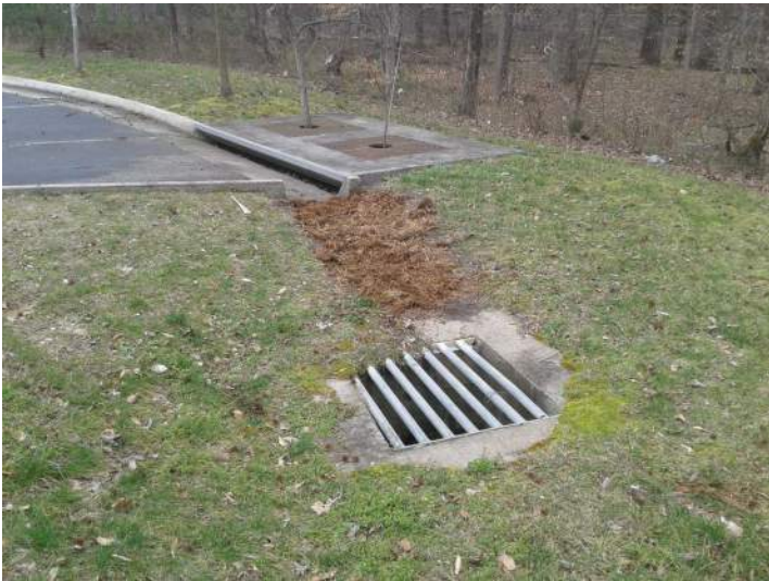
Seed and straw installed
