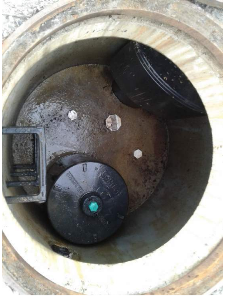
35 after pressure wash and vac.
