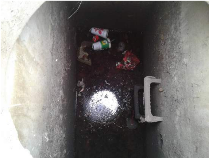
Before. Chamber 1 of unit 31.
