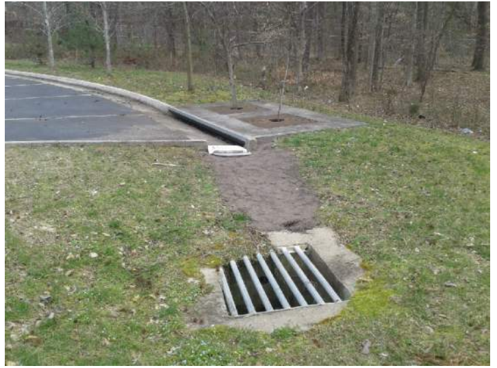
Filled erosion area with topsoil
