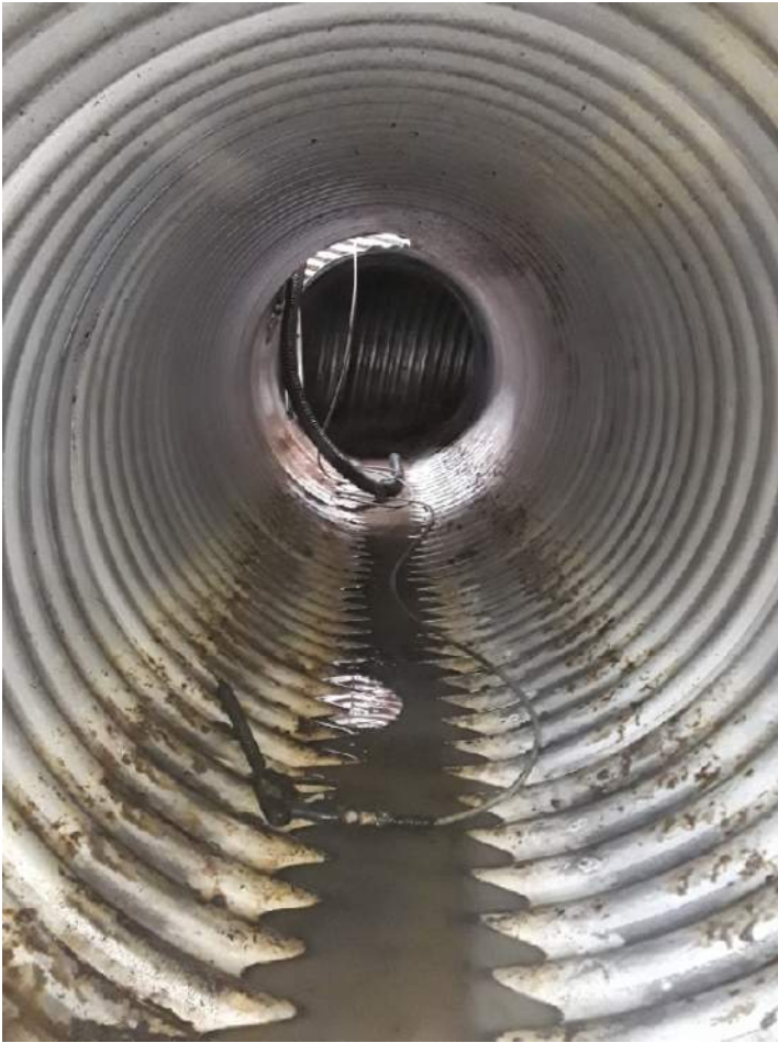
CMP 15 after. Removed 800 gal
