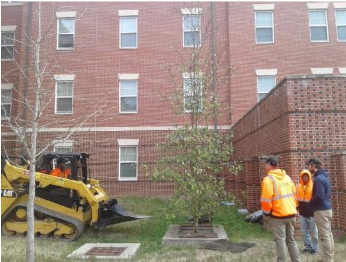
Unit 19 removing tree.
