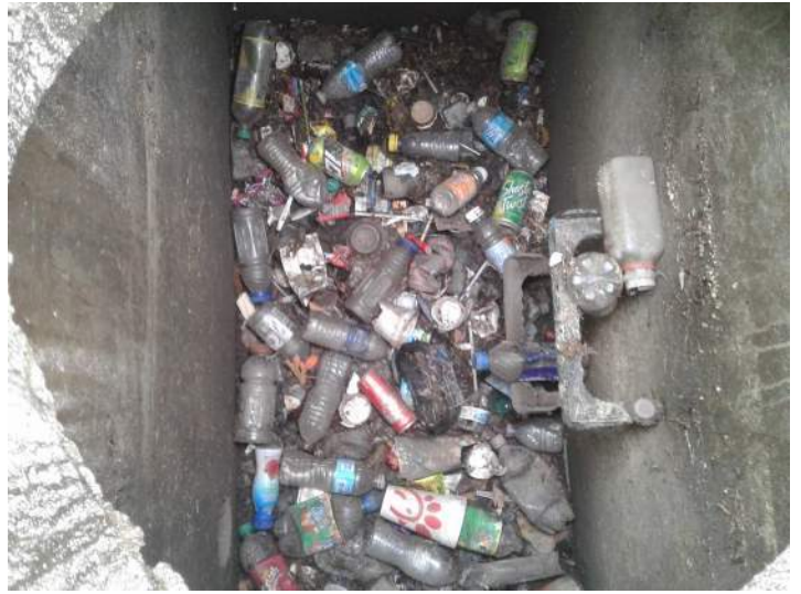
Before. Unit 31 chamber 2.
