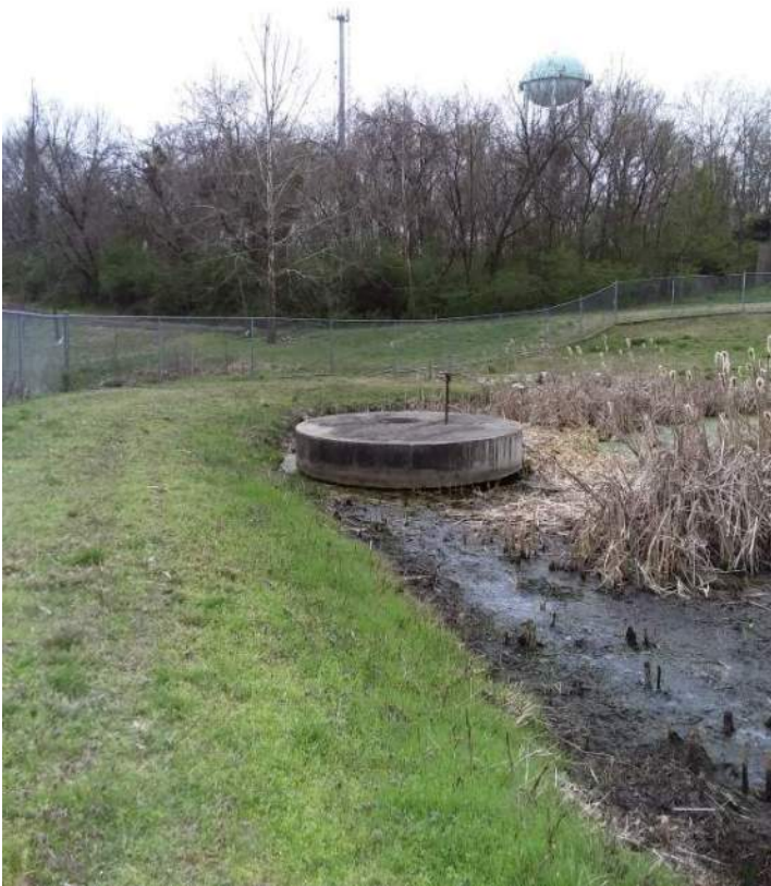
BMP 30: showing location of outfall structure near rip rap emergency spillway
