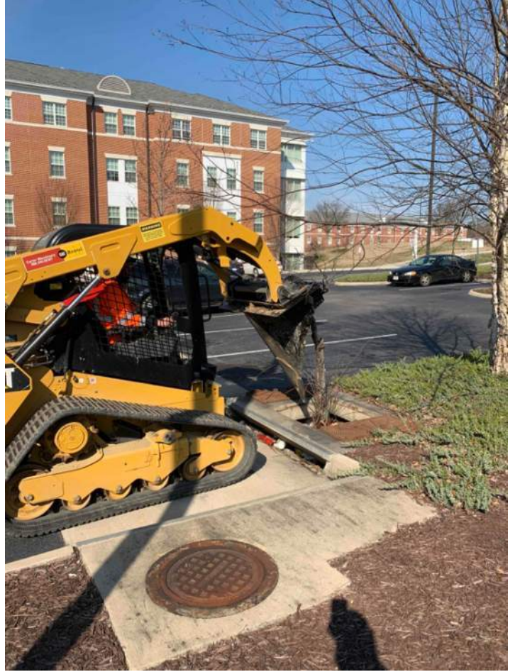
Unit 7 tree removal
