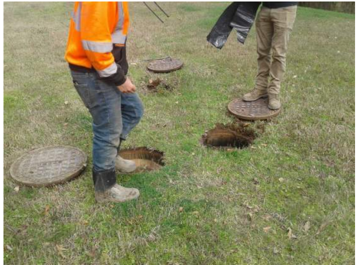
Opening up unit 31.
