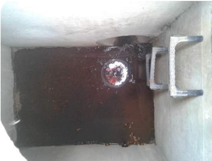
Unit 31 chamber 3. No debris to remove.
