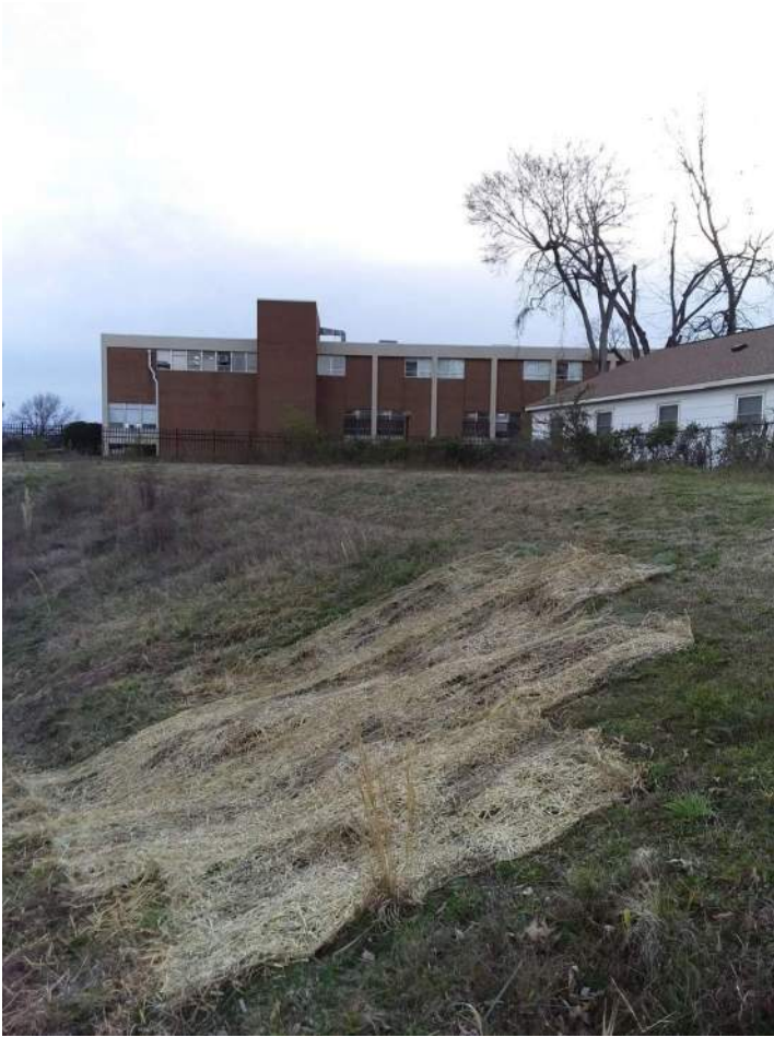
BMP 46: Different angle of the same repaired section.
